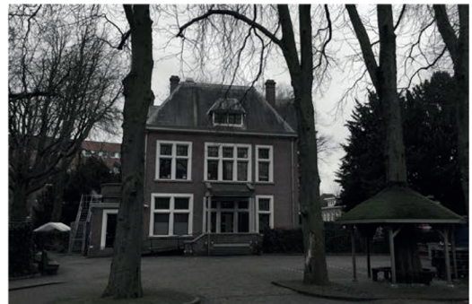
Image 28: The grounds and drop-in at Ripperdastraat
